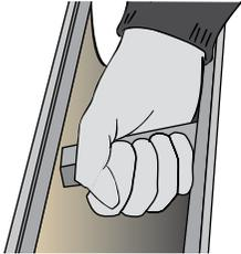
2. **To install grate**, align the anti-shunt lugs on the underside edge of the DrainLok grate with the recesses in the channel rail, or align the QuickLok spigot directly over locking bar. Push down or stand on grate until it clicks into position.
