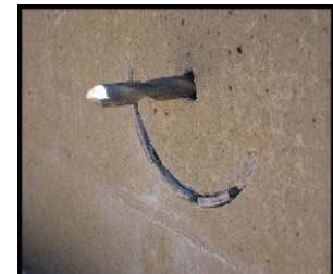
Figure 6 Wet drilling recommended.
