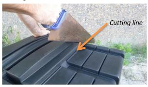
Flip the top section upside down and trace the base profile onto the bottom of the top section. Enlarge the hole with a jig saw. This will allow the base section to slide inside the top section. The marking can be done before cutting if desired.
