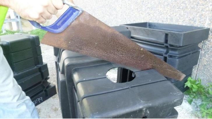
3. Fit the pit base underneath the existing conduit. Cut conduit flush with the inside of the pit if required.
