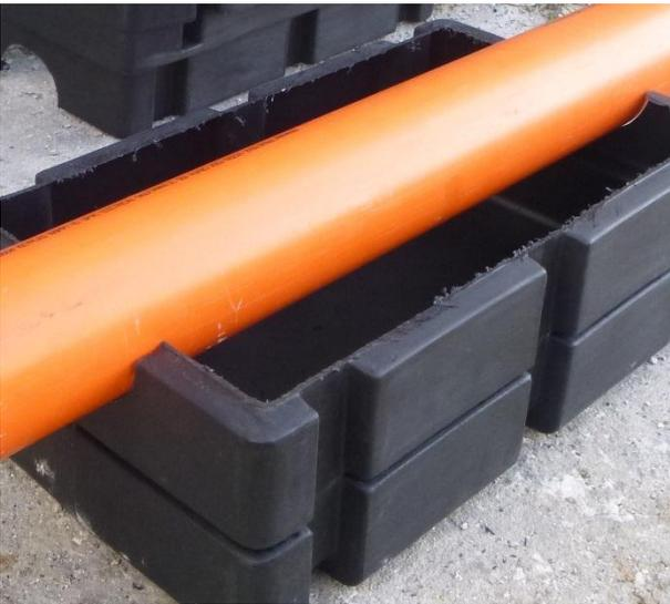
4. Fit top section of pit over the pipe and align with pit base. Ensure the top of the pit is installed at the required finished floor level.
