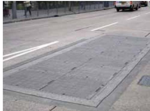
between the covers widthways, the cover profiles are both undercut and therefore require an additional centre frame to provide the seal and a support beam to take the loadings
